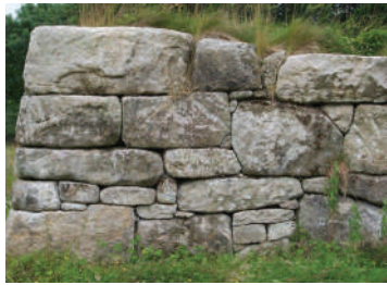
Fig. 1.11: Dry rubble masonry
