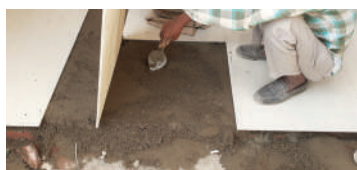
Step 2: Pasting of mortar
