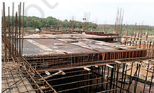
Fig. 4.4 (a): Shuttering for beam and RCC Floor
