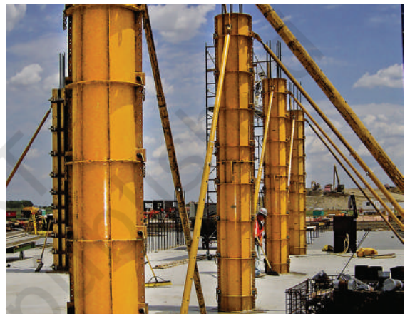
Fig. 4.2: Formwork for circular columns
