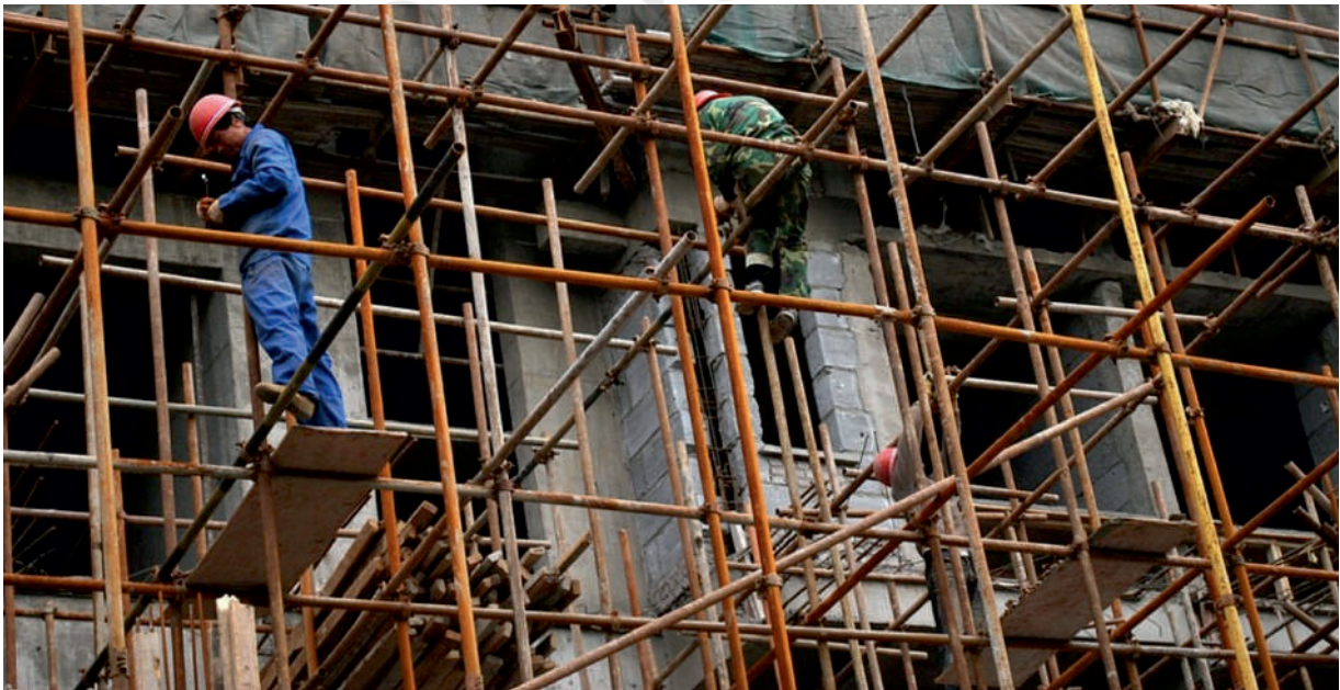
Fig. 3.1: A view of Scaffolding
