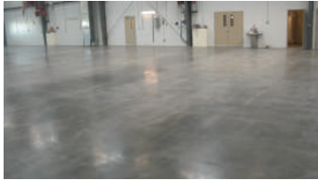
Fig. 5.4: Cement concrete flooring
