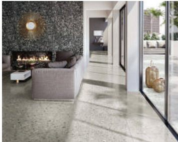
Fig. 5.6: Terrazzo tile flooring
